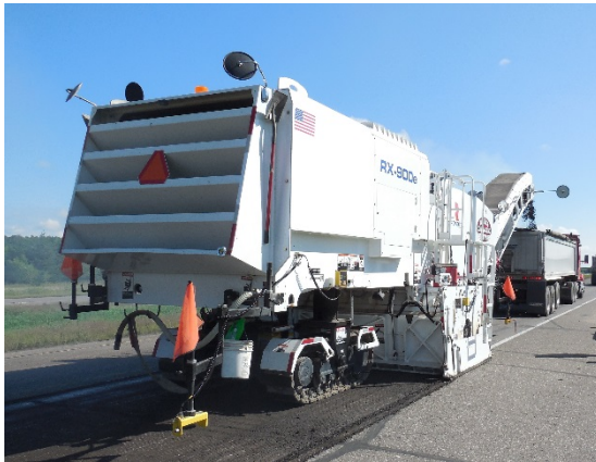
Step 1. Micro mill is performed across the entire lane width.
