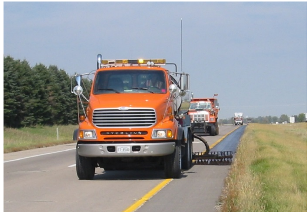
Step 2. Fog seal is applied to pavement surface. The example above shows a fog seal applied to a bituminous shoulder.
