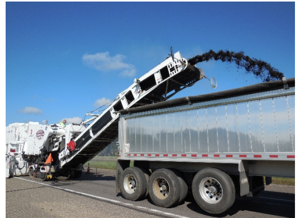
Step 2. Millings are collected by a haul truck.
