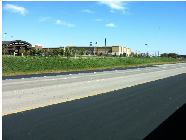
Step 3. Fog Seal must be allowed to cure.
