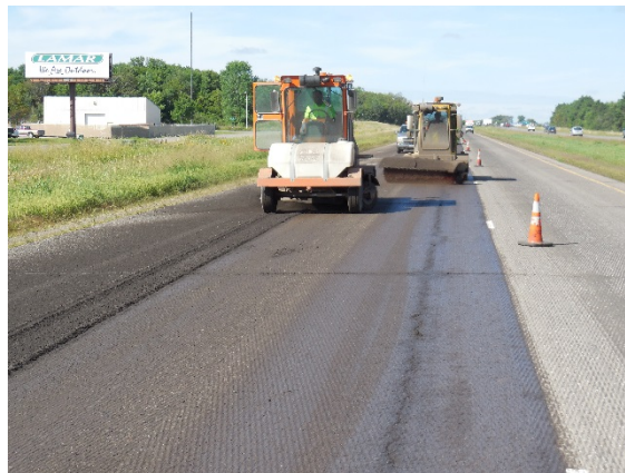
Step 3. Milled surface is swept free of debris.
